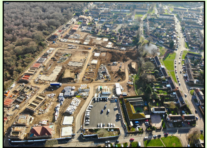
Above: Tadworth Gardens construction site 2019. Chetwode Road just visible at bottom.
