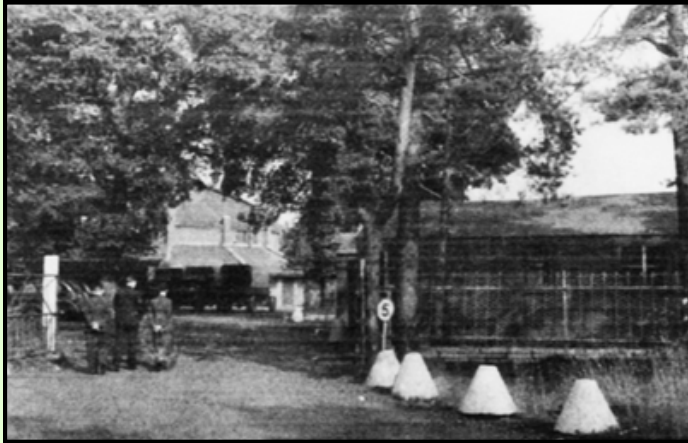
The buoys being used as verge protectors outside WW2 army depot, Burgh Heath. Now the ASDA shop.
