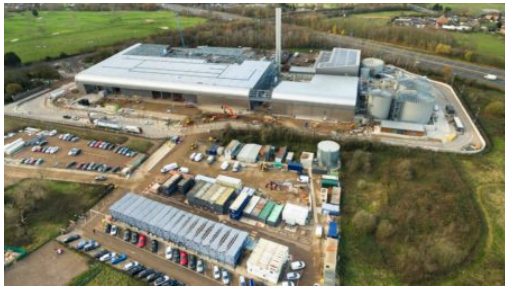
The Suez Surrey Eco Park Facility in Shepperton
